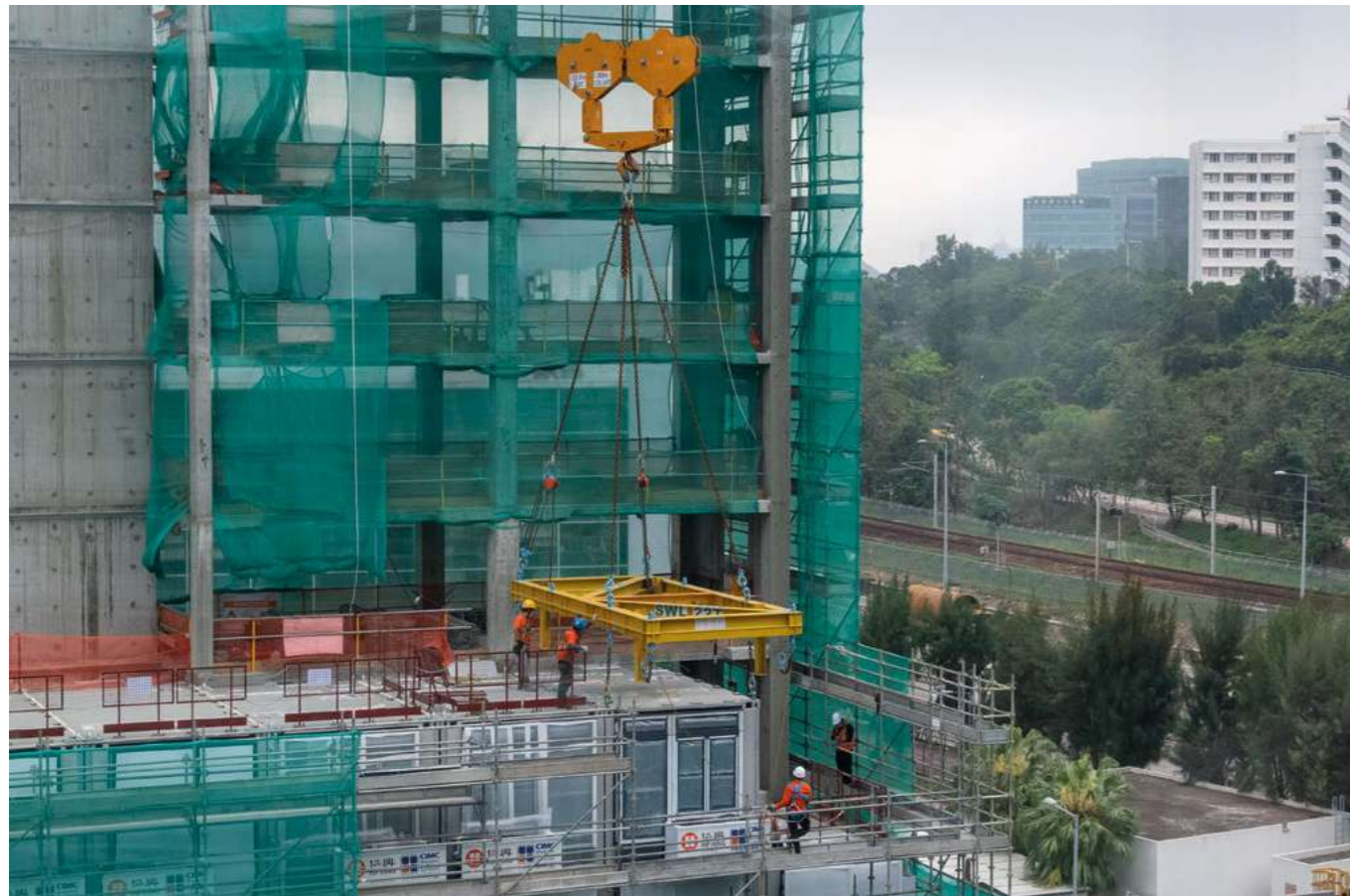
Modular Integrated Construction on-site installation
